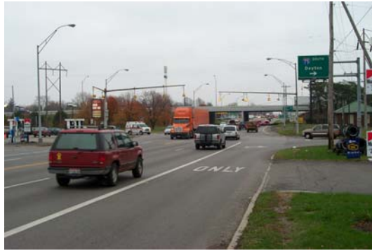
Eastern approach to the interchange
